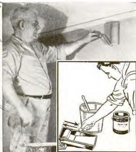
Cloth-covered roller is "loaded" in flat-bottom pan
